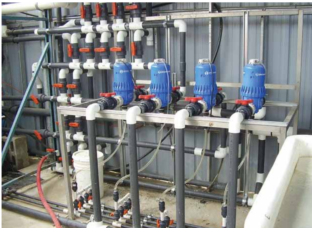
Using a main filter on the incoming water will protect the fertilizer injectors.
